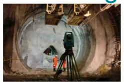
Surveying and monitoring systems made the construction of the Gotthard Base Tunnel in the Swiss Alps possible. The tunnel will be inaugurated on 1 June 2016 and the breakthrough on 15 October 2010 was due to highly precise surveillance and monitoring technology. The 57km long tunnel (35.4 miles) is the longest and deepest rail tunnel in the world
