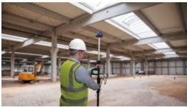
Racelogic has launched a brand-new indoor positioning system, called VIPS, which is an advanced system for measuring real-time 3D position to an accuracy of ±2cm in areas where GPS is not available. This makes it an ideal tool for construction applications both indoors and in urban areas. The system has been designed for any application that requires accurate measurement and recording of 3D positioning. It enables GPS-based technologies to operate in GPS-denied environments.
