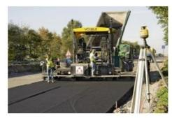
Topcon and TSD Integrated Systems, a joint venture of Topcon and supplier of electrohydraulic equipment, Sauer Danfoss, have unveiled Millimeter GPS precise positioning technology for the paving industry, creating a 3D-GPS+ control system for pavers, profilers and trimmers
