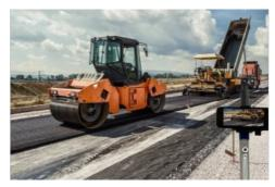
MetaSpatial Solutions' new platformagnostic SmartSurveyor system turns any smartphone (iOS/Android), tablet or low-cost consumer-grade drone into a precise mapping system with 2cm mapping accuracy in XYZ. MetaSpatial Solutions is an Australian-based geospatial and mapping technology company.
