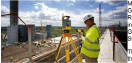
Maidenhead-based civil engineers, Costain, have purchased a combination of Trimble R8 GNSS receivers and Trimble S6 robotic total stations for use on the Riverside Resource Recovery Facility currently under construction at Belvedere in South-East London. These instruments will help Costain to deliver the main buildings, jetties, roads and offices for the GBP350 million project which is being developed by Cory Environmental and built by Swiss plant construction company Von Roll Inova.
