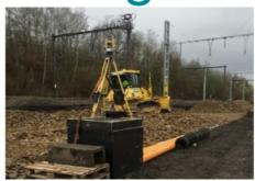
Advanced total station solutions from Topcon Positioning were chosen to support a project to renew the railway switches and crossings at a site in Belgium. By providing accurate real-time data, the total stations helped guide the machinery to ensure efficiency, safety and quality during the project.
