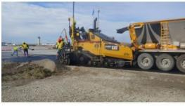
Trimble has introduced the Trimble Roadworks 3D Paving Control Platform for Asphalt Pavers, the next-generation platform for 3D asphalt paving control systems. Trimble Roadworks is a highly accurate, automatic 3D screed control system that can significantly improve paving productivity and rideability by directly referencing the design rather than a surface or stringline to minimize asphalt usage, reduce waste and overruns and finish projects on time and under budget.
