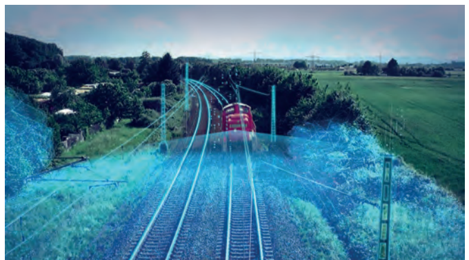
▲ The data collection process is built around a Trimble MX9 mobile mapping system that can be installed on trains, trolleys and cars, as needed. (Image courtesy: Siemens Mobility)
