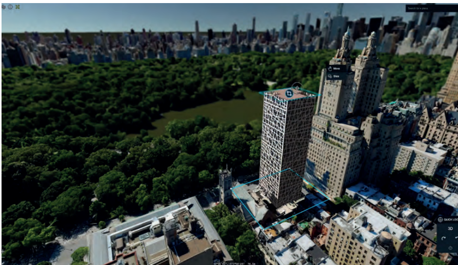
▲ Scenario 3: A digital twin used in planning the construction of a high-rise building. (Image courtesy: Hexagon)
