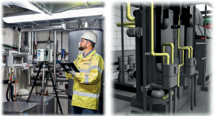
▲ Capturing assets with precision through Scan-to-BIM. (Image courtesy: Murphy Geospatial)
