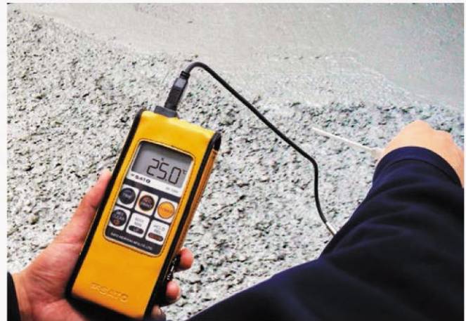
Measuring concrete temperature (SK-1260 with soft pouch)
