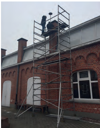
▲ CORS installation in Ruiselede, Belgium.
